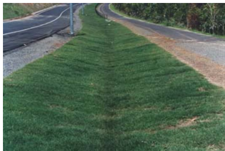
Typical use of turf in a concentrated flow environment
