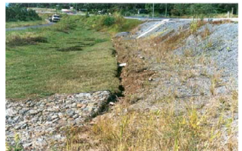
Poorly installed and maintained reinforced turf showing erosion along the turf/soil interface and weed invasion of the turf grasses
