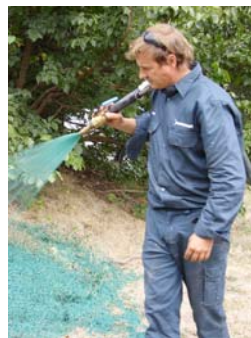
Aquaseeding demonstrating hydromulching.
