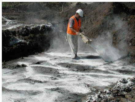
Treating acid sulfate soils with lime prior to use as a construction material.
