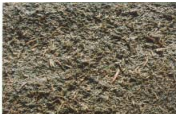
Close up photo of a recently applied cane and paper BFM. Note the 100% soil surface coverage of the BFM.
