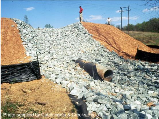
**Photo 11 – Emergency spillway located within the fill embankment**
