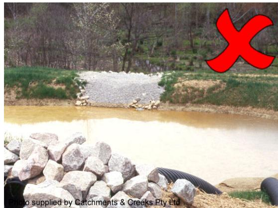
**Photo 16 – Spillway crest with inadequate depth or profile**
