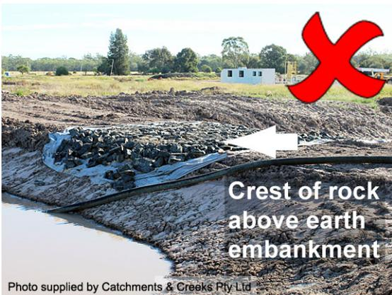
**Photo 15 – Spillway rock protection sits above the embankment height**
