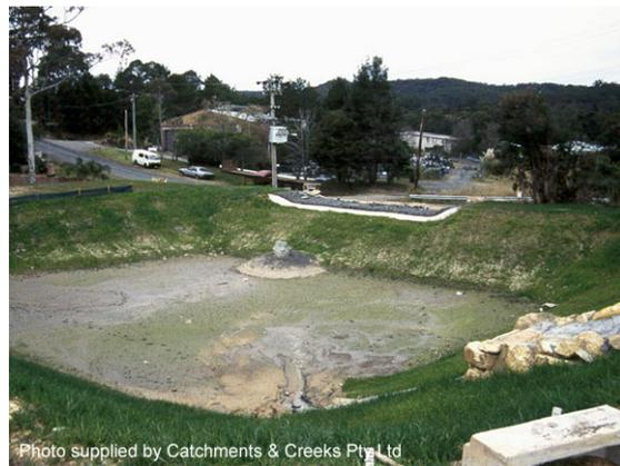
**Photo 14 – Rock-lined spillway—note concrete sealing of the spillway crest**
