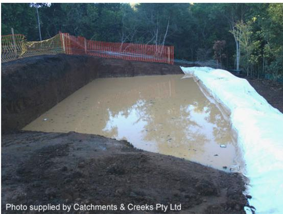
**Photo 13 – Fully recessed basin with natural ground forming the spillway**
