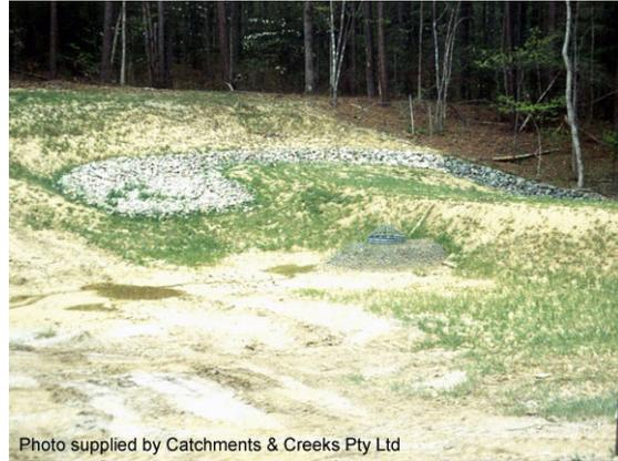
**Photo 12 – Emergency spillway located within virgin soil to the side of the embankment**
