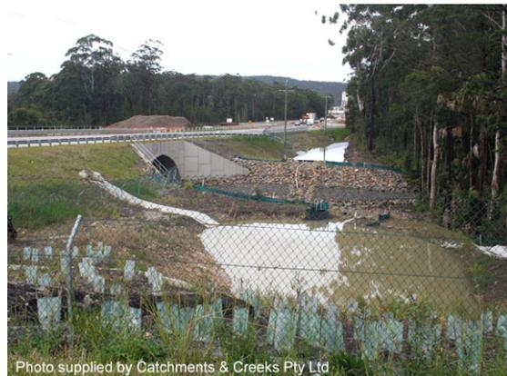
Photo 21 – Sediment basins converted to permanent stormwater treatment ponds on highway project
