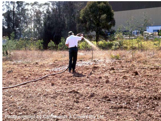
Photo 16 – Hydraulically applied blankets
