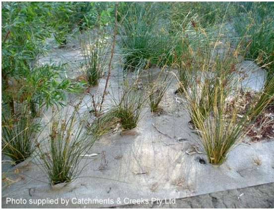
Photo 13 – Erosion control blankets
