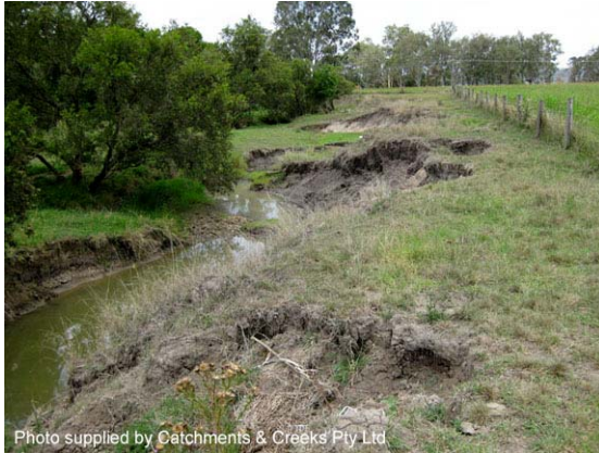
Photo 9 – Lateral bank erosion
