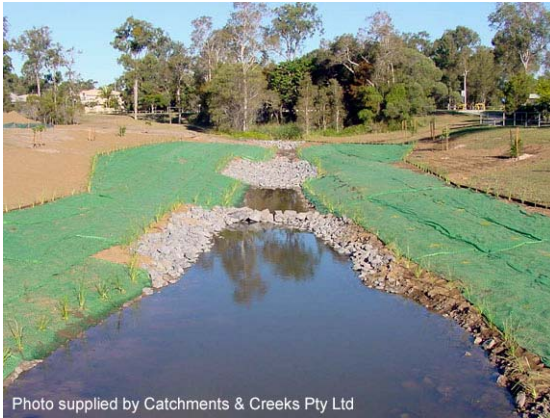
Photo 1 – Erosion control blankets installed during channel revegetation
