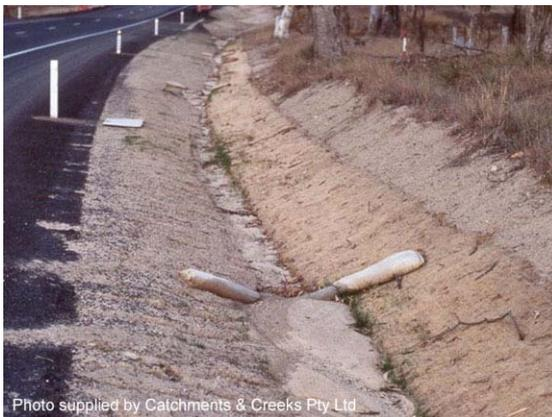
Photo 1 – Sandbag check dam sediment traps
