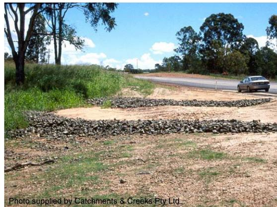
Photo 2 – Rock check dam sediment traps
