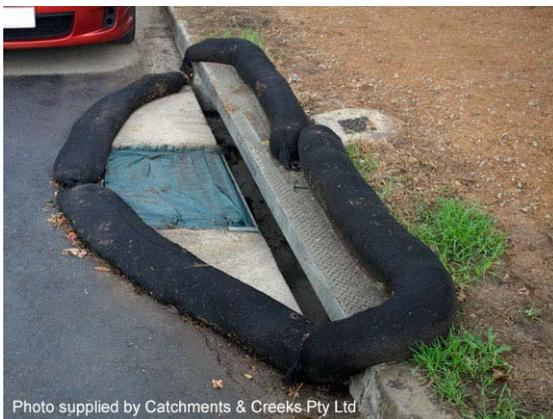
**Photo 1 – Filter socks used to form a 'sag' inlet sediment trap**
