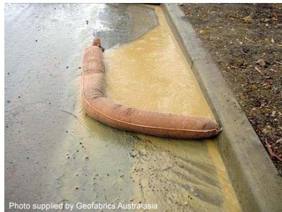
**Photo 2 – Filter socks used to form an 'on-grade' kerb sediment trap**
