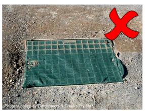
Photo 2 – Shade cloth should <u>not</u> be used, also note no sediment collection trench formed around the drop inlet
