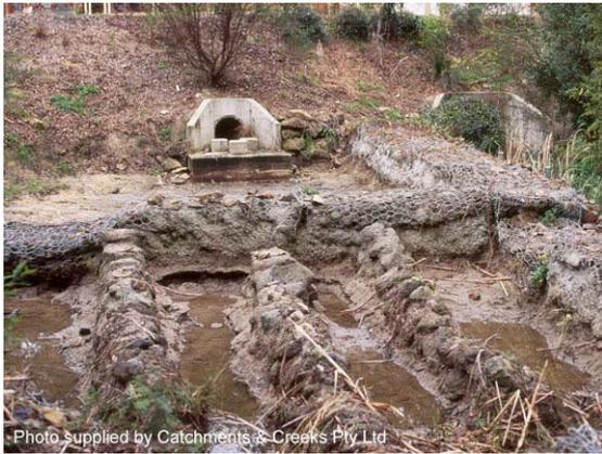
Photo 11 – Outlet sediment trap during construction phase
