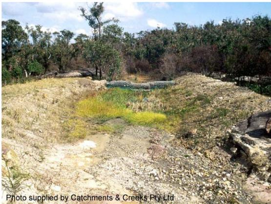
Photo 13 – Coarse sediment trap collecting sediment from road discharge
