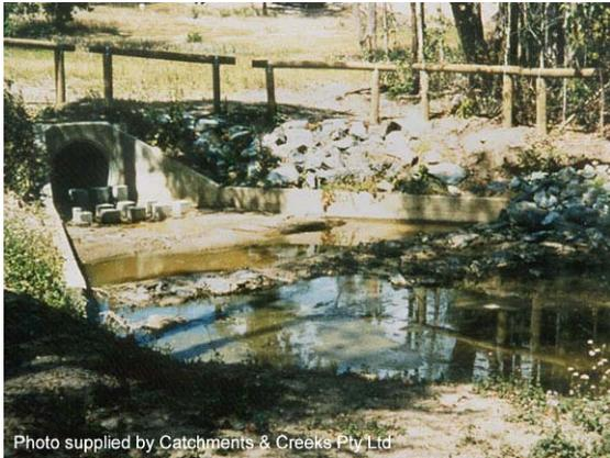
**Photo 1 – Excavated sediment trap just prior to scheduled clean-out (note energy dissipater at end of pipe)**
