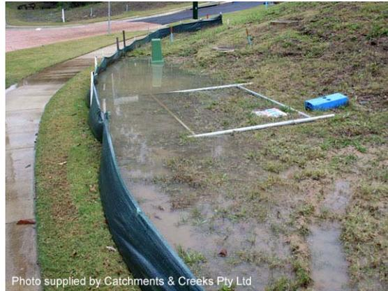
Photo 2 – Sheet flow approaching a sediment fence
