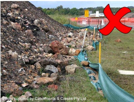
**Photo 31 – Damage by shifting fill**
