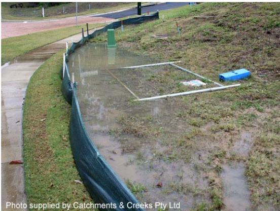
**Photo 9 – Sediment fence placed along the contour**
