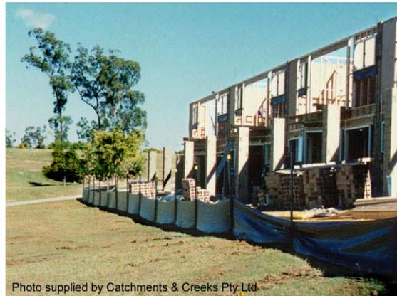
Photo 2 – Sediment fence located down-slope of multi-dwelling building site
