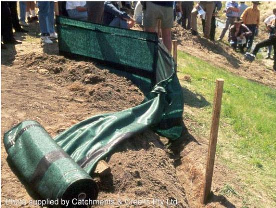
Photo 1 – Installation of a sediment fence
