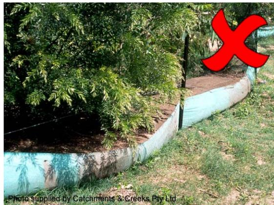
**Photo 34 – Sediment not removed after storm**
