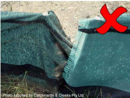
**Photo 19 – Inappropriate junction**
