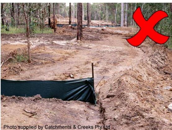
**Photo 35 – Flow allowed to bypass the fence**
