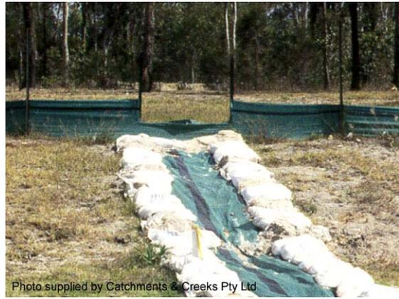
Photo 38 – Spill-through weir with outlet chute
