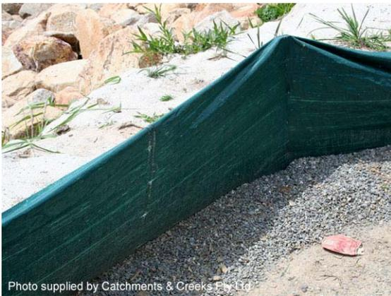
**Photo 15 – Bottom of fabric buried under aggregate**
