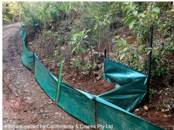
**Photo 12 – Alternative design of a fence 'return'**
