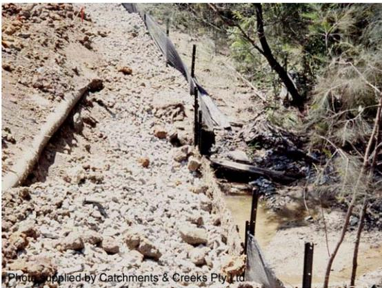
Photo 39 – Spill-through weir with up-slope aggregate filter
