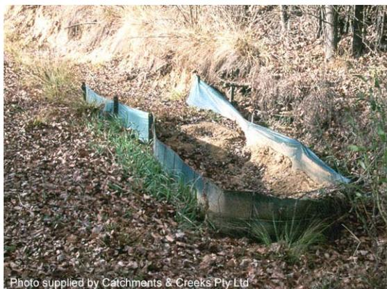
Photo 1 – U-shaped sediment trap
