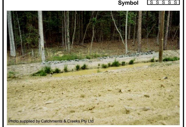
Photo 1 – Sediment trench located at the base of a fill batter on a road construction project (USA)
