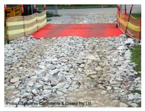
Photo 1 – Vibration grid and rock pad
