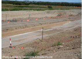
Photo 6 – Wash bay operating as a dry vibration grid during dry weather
