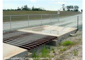
Photo 5 – Vibration grids are usually located prior to a wash bay
