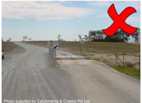
Photo 8 – Dividing site entry and exit lanes can result in vehicles bypassing the construction exit
