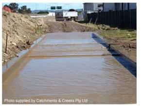
Photo 1 – Automated wash bay located on Photo 2 – Temporary wash bay located on a road construction project
