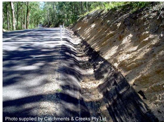
**Photo 12 – Roadside catch drain lined with an erosion control mat sealed with bitumen**
