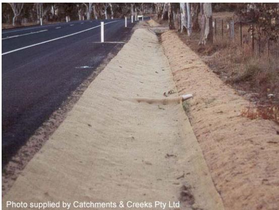
**Photo 11 – Roadside table drain lined with a temporary jute erosion control mat**
