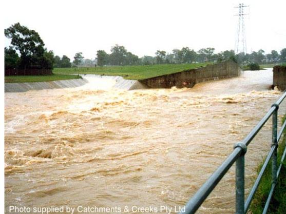
Photo 6 – Hydraulic jump dissipater downstream of detention basin outlet
