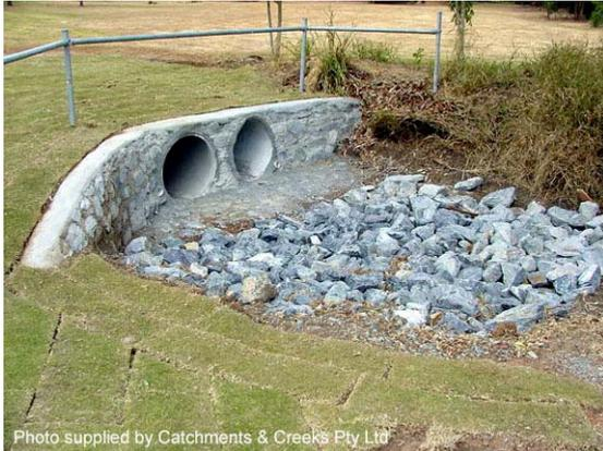
Photo 3 – Rock pad outlet structure
