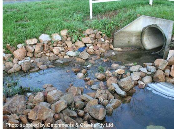
Photo 4 – Rock pad outlet structure
