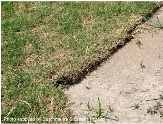
Photo 3 – Example of up-slope edge of turf that can redirect water flow
