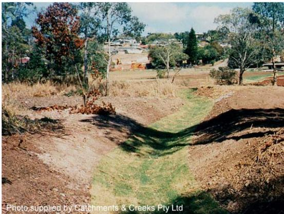
Photo 1 – Grass-lined flow diversion channel
