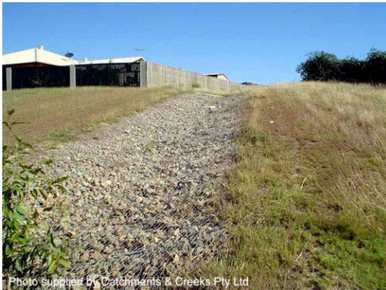
**Photo 1 – Rock mattress-lined drainage chute**
