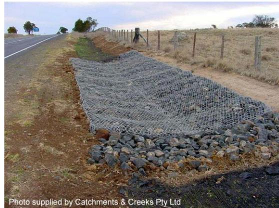
**Photo 2 – Rock mattress-lined table drain (stormwater infiltration pit)**
