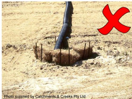
**Photo 10 – Inappropriate flow release**
