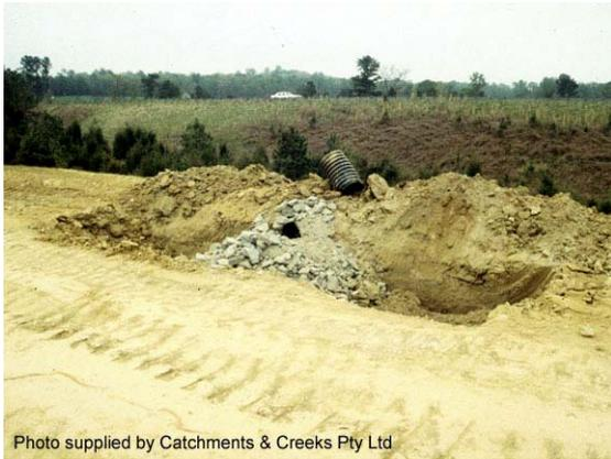
**Photo 5 – Inlet sediment trap**
