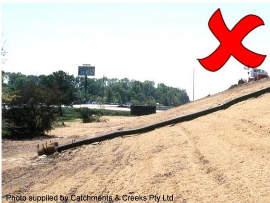
**Photo 9 – Inappropriate flow release**
