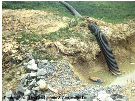
**Photo 8 – Outlet sediment trap**
