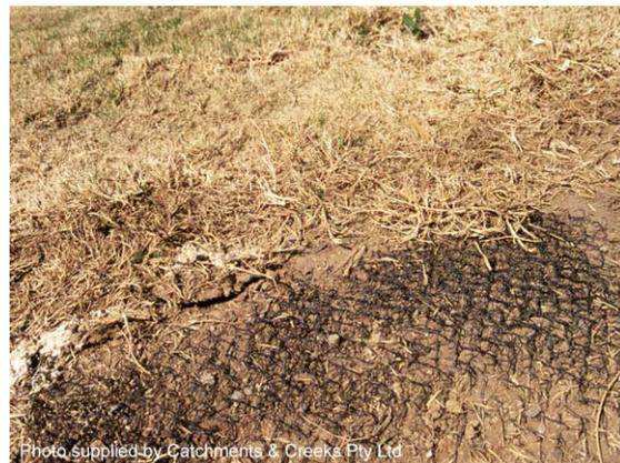
**Photo 2 – Reinforced grass with the grass layer removed as part of a field day demonstration**
