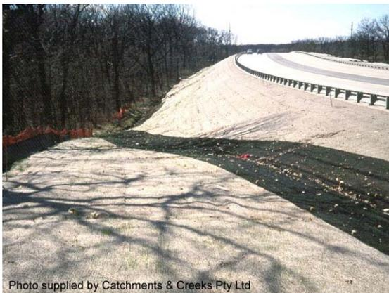
**Photo 1 – Permanent turf reinforcement mat (black) surrounded by temporary erosion control blankets**
