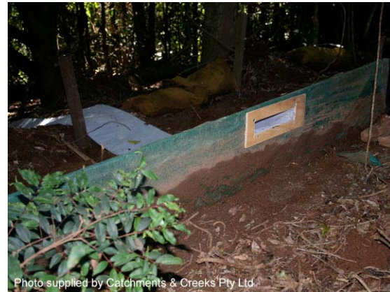
Photo 2 – Note filter tube inlet is raised above ground level to encourage ponding
