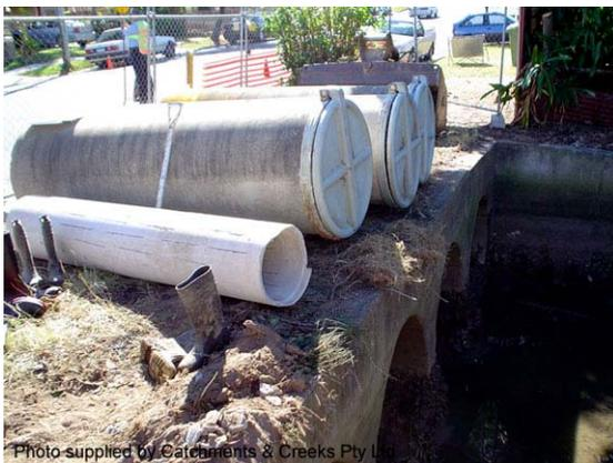
**Photo 3 – Flood bypass pipes with attached tide gates prior to their installation shown right**
