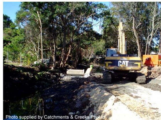
**Photo 4 – Installation of downstream cofferdam with flood bypass pipes (left) within a tidal waterway**
