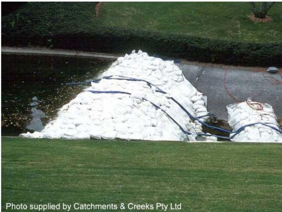
**Photo 1 – Upstream sandbag cofferdam located within a concrete channel during channel maintenance**
