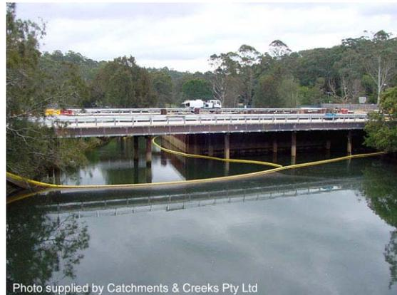
**Photo 2 – Sheet piling used to form a dry work area with a floating silt curtain used as a sediment containment system**
