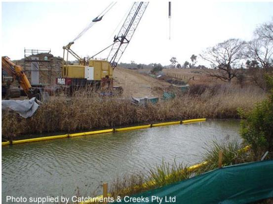
**Photo 1 – Silt curtain used as an isolation barrier**
