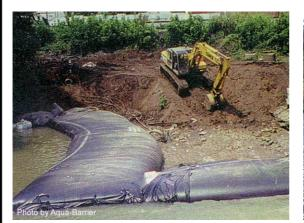
Photo 1 – 'Aqua Barrier' inflatable isolation barrier
