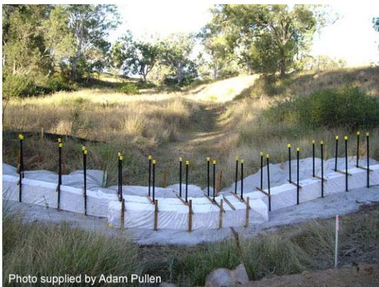
Photo 1 – Modular sediment barrier
