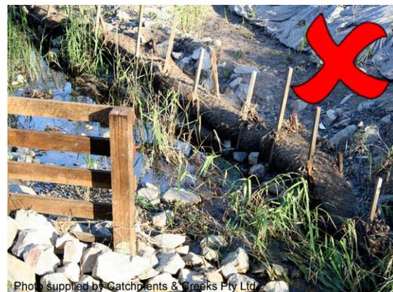
Photo 4 – Significant bank erosion adjacent the geo logs (note, stakes sit too high above top of logs)
