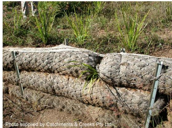
**Photo 2 – Geo logs placed on the outside of a channel bend**
