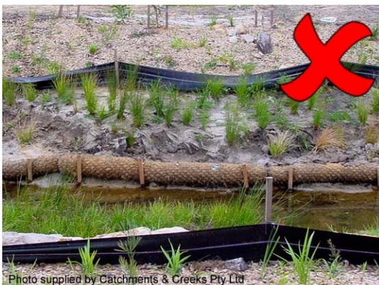
Photo 3 – Significant bank erosion adjacent the geo logs (note, stakes at correct height, but wrong spacing)
