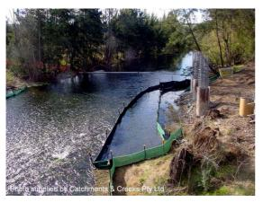
Photo 1 – Sediment fence isolation barrier with landward sediment fence
