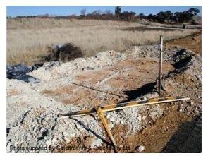
Photo 1 – Washing-out a concrete truck
