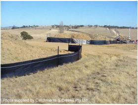
Photo 2 – Sediment fence placed downslope of soil stockpile
