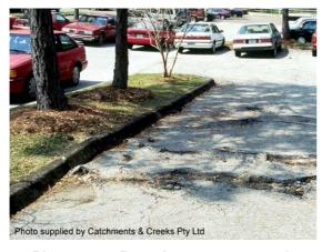
Photo 11 - Root damage to car park pavement
