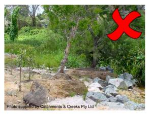
Photo 9 – Recent earthworks have left this protected tree elevated well above the surrounding ground level
