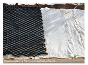
Photo 7 – Placement of filter cloth might not always be required
