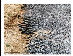
Photo 1 – Cellular confinement system used to restrict gravel movement on a permanent car park
