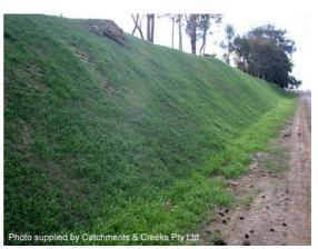
Photo 6 – Grass establishment on steep slope
