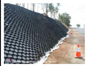
Photo 5 – Installation of matrix on a road cutting
