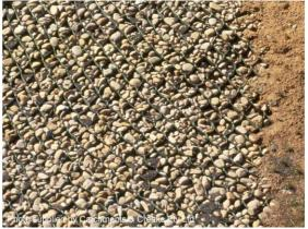
Photo 8 – Cellular confinement system used to hold aggregate on an embankment
