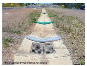
Photo 5 - Check dam sediment traps
