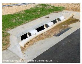
Photo 3 - 'Sag' inlet sediment trap
