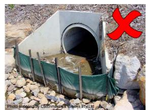
Photo 9 – Sediment should <u>not</u> be allowed to collect within the pipe
