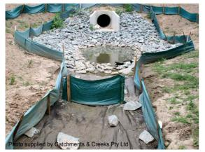
Photo 5 – Pipe outlet sediment trap
