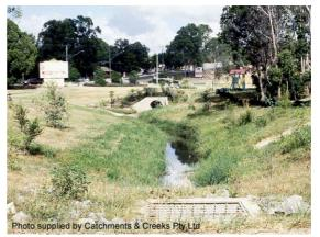
Photo 8 – Temporary conversion of an outlet swale into a sediment basin
