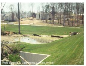
Photo 4 - Coarse sediment trap
