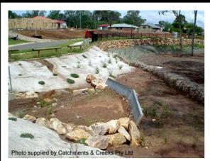
Photo 3 – Note temporary gabion wall
