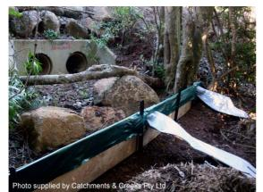
Photo 7 – Filter tube dam placed downslope of stormwater outlet
