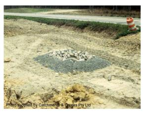
Photo 1 – Rock and aggregate drop inlet protection located with dual carriageway
