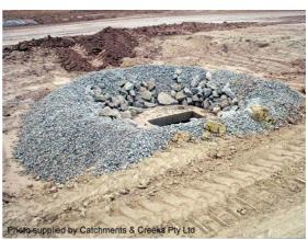
Photo 2 – Rock and aggregate drop inlet protection
