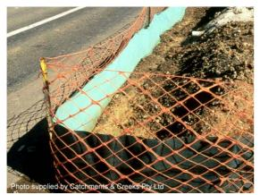
Photo 25 – Installation with safety fencing used as support
