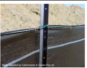
Photo 22 – Installation with top wire support
