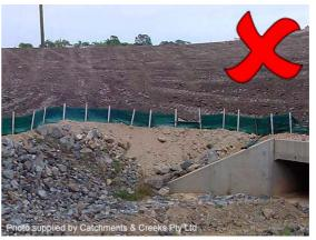
Photo 36 – Spill-through weirs must not discharge onto unstable land
