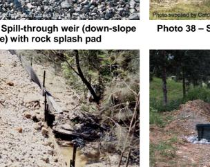
Photo 39 – Spill-through weir with up-slope aggregate filter
