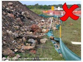
Photo 31 – Damage by shifting fill
