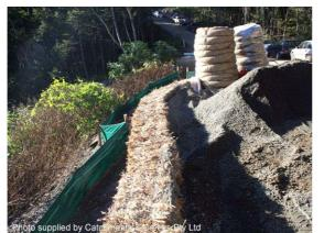
Photo 7 – Use of straw bales to prevent direct contact of stockpiles with the fence
