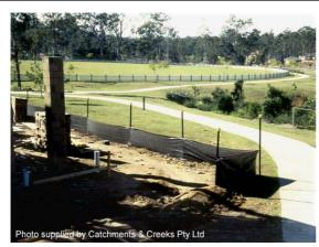
Photo 21 – Installation without backing weir/mesh
