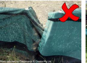
Photo 19 – Inappropriate junction
