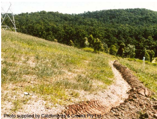
Photo 7 – Earth-lined catch drain
