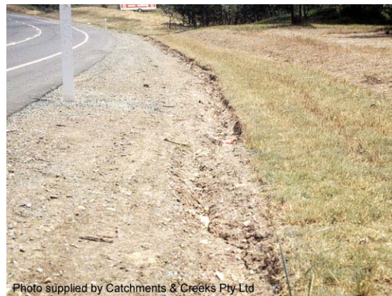
Photo 10 – Common erosion problem resulting from flow bypassing along up-slope edge of turf
