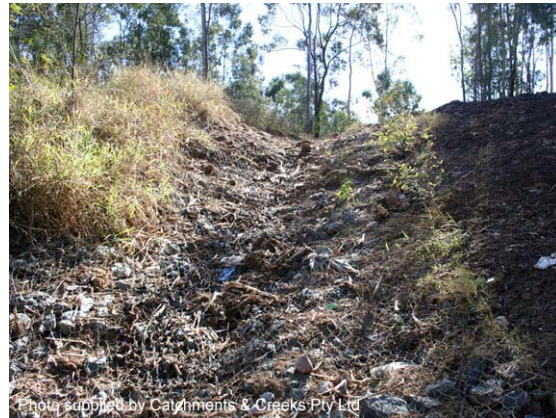
Photo 16 – Partially vegetated, rock mattress-lined batter chute
