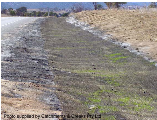
Photo 1 – Temporary jute mesh with emerging grass
