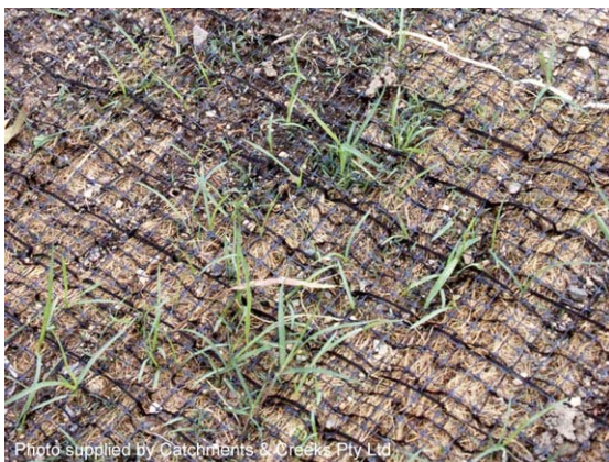
Photo 10 – Synthetic root reinforcing with organic mulch layer
