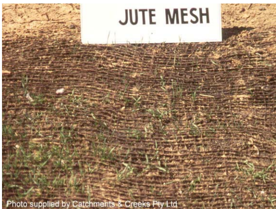
Photo 12 – Jute mesh is effectively an organic mat reinforcing
