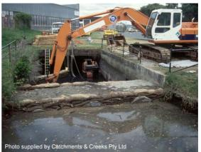
Photo 2 – Downstream sandbag and compacted fill cofferdam located within a storm drain during drain maintenance
