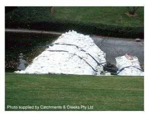
Photo 1 – Upstream sandbag cofferdam located within a concrete channel during channel maintenance
