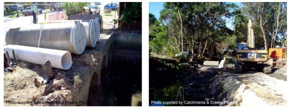
Photo 3 – Flood bypass pipes with attached tide gates prior to their installation shown right
