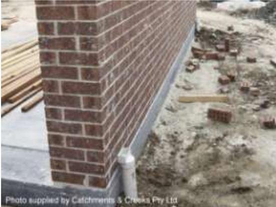
Permanent sub-surface drainage installed
