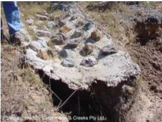
**Tunnel erosion under concrete drain**
