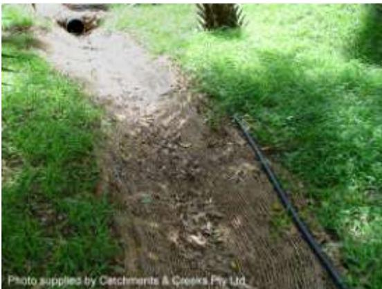
Stormwater drain lined with jute mesh
