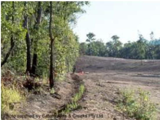
**Catch drain formed up-slope of work site**
