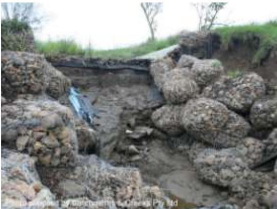
**Failed gabion overflow spillway**
