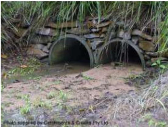
**Sedimentation of drainage pipes**
