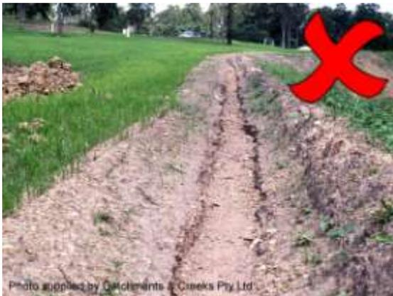
Erosion of an open soil drain
