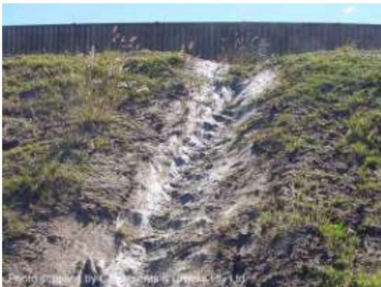
Geotextile-lined drainage chute
