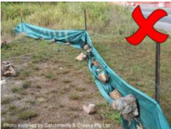
Toe of fabric incorrectly anchored
