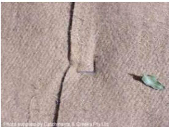
Temporary (jute) erosion control blanket
