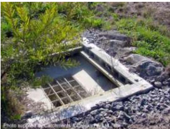
Block & aggregate drop inlet protection
