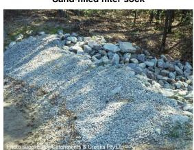
Rock filter dam with aggregate filter
