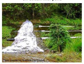
Instream rock filter dam with filter tubes
