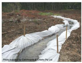
Temporary drain lined with filter cloth
