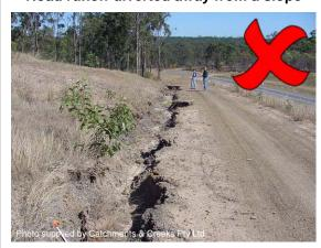
Batter drain cut into a dispersive soil
