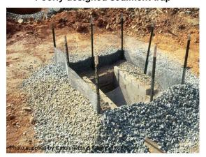
Mesh and aggregate drop inlet protection
