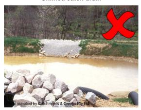
Poor sediment basin spillway design
