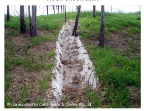
Batter chute lined with filter cloth
