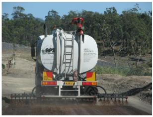
Bitumen based geobinder 'PetroTac' being applied to a mining haul road
