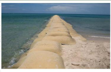
The ELCOROCK® shoreline protection system from Geofabrics Australasia Pty Ltd (Geofabrics) is being applied to address the coastal foreshore erosion and management.
