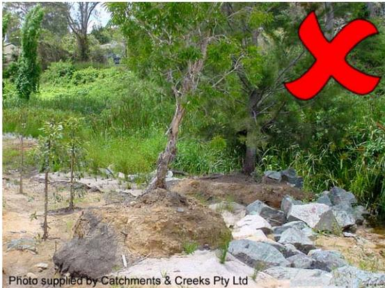
**Photo 9 – Recent earthworks have left this protected tree elevated well above the surrounding ground level**
