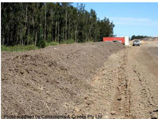
**Photo 5 – Mulch berm produced by tub-grinding cleared vegetation**
