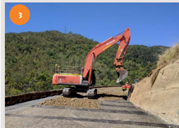
A 300MM LAYER OF AMELIORATED SUBSOIL WAS USED AS SUITABLE GROWTH MEDIA
