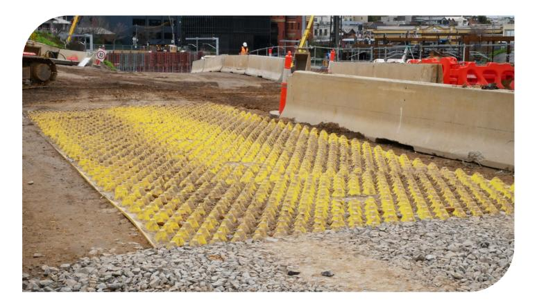
To the delight and with some surprise to some the FODS installation proved to not only work well as intended but demonstrated its robustness when the team on site had no choice but to run a steel cleat digger and an 80 tonne cleated piling rig across the mats.
