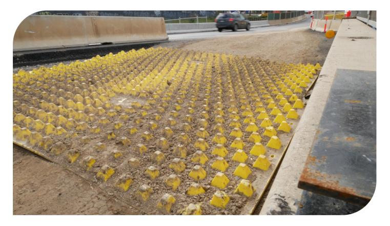
Subsequently, additional FODS were acquired by the project, with one site noting that the FODS work more effectively than traditional rumble grids. The site have both measures in place with exiting traffic first running over the rumble grid and then the FODS. In this scenario the FODS are capturing a great deal of material that the rumble grid is failing to remove.
